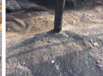
2. Seal barrier directly to VaporStake™
