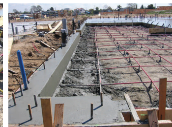
5. Permanently leave the lower portion of VaporStake™
