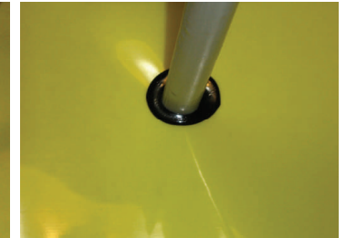
3. Properly align the nail holes and drive the VaporStake™ through the StegoWrap®. The VaporStake™ can be turned while the mastic is wet, but do not turn it after the mastic has set up.
