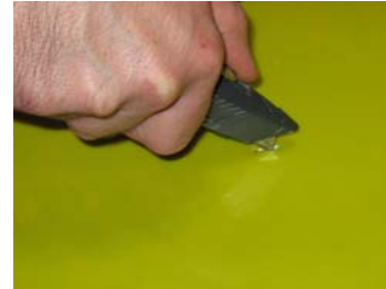
1. If necessary, use a utility knife to puncture a slit in the vapor retarder. The slit should be no larger than the diameter of the VaporStake™ being used.
