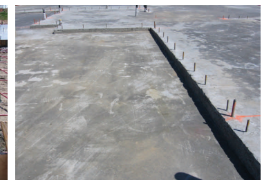
6. Finish slab over VaporStake™
