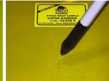
2. Dip the pointed end of the VaporStake™ into the mastic that is provided by the vapor retarder..
