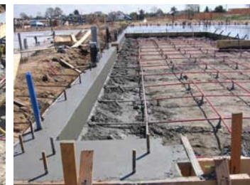
5. Permanently leave the lower portion of VaporStake™
