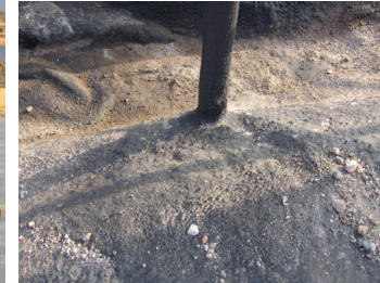
2. Seal barrier directly to VaporStake™
