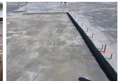
6. Finish slab over VaporStake™
