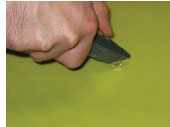
1. If necessary, use a utility knife to puncture a slit in the vapor retarder. The slit should be no larger than the diameter of the VaporStake™ being used.
