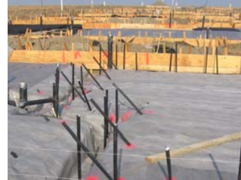
1. Using a sledge hammer, drive VaporStake™ into ground
